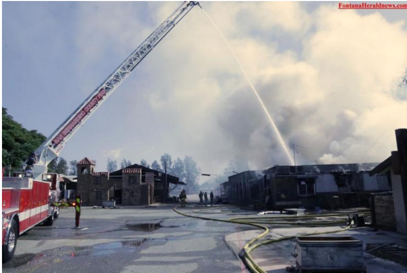
A fire damaged two buildings in southwestern Fontana on the morning of Nov. 13 (Contributed photo by Connie Caruthers)
