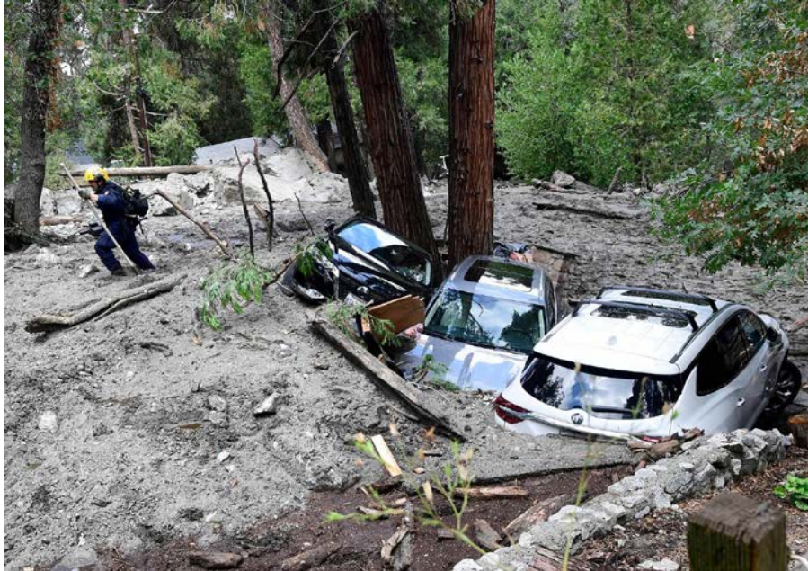
A search and rescue member walks through thick mud as they search a flood-destroyed home on Prospect Drive in Forest Falls on Tuesday, Sept. 13, 2022. Large mud flows hit the area Monday afternoon after a large thunderstorm hit the area heavily damaging at least 4 homes. (Photo by Will Lester, Inland Valley Daily Bulletin/SCNG)
