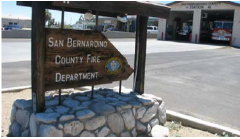
One of two San Bernardino County Fire Department stations in Yucca Valley
