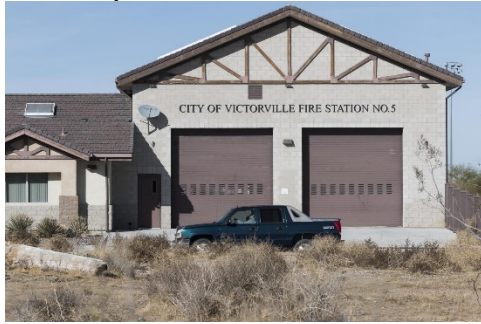
Victorville Fire Department Station 315 on Eucalyptus Street in an updated photo. Daily Press File Photo
